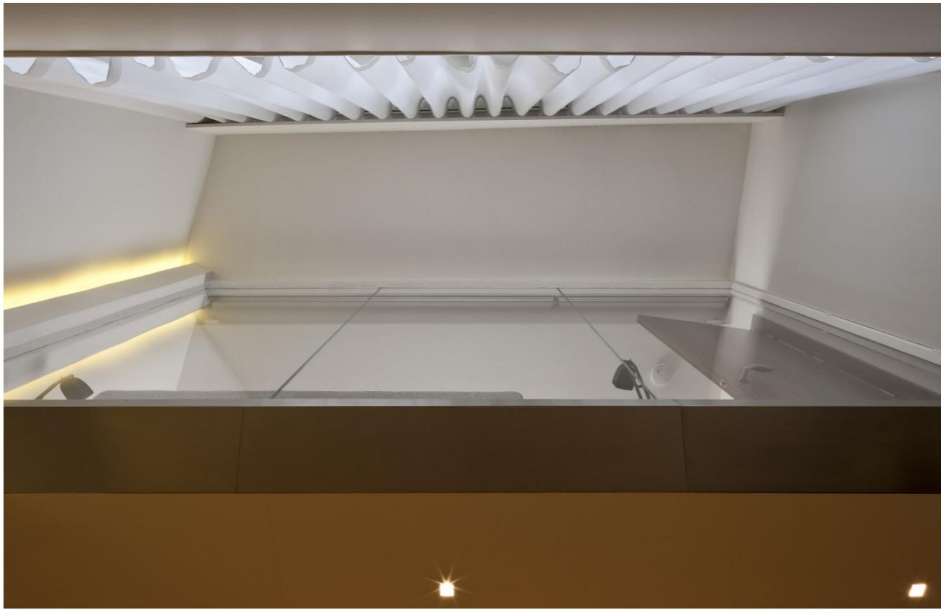
A new study/ living room was created on the ground floor through the insertion of a new floor structure within the double-height basement dining room. The new floor structure is set away from the front elevation's sash windows so that these carry on in providing light and ventilation to the basement dining room via a light slot.
